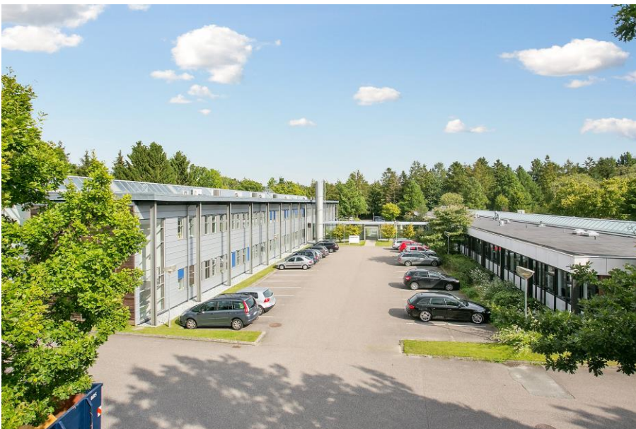
Fig. 1. TOOsonix Facility in Hørsholm, Denmark.
